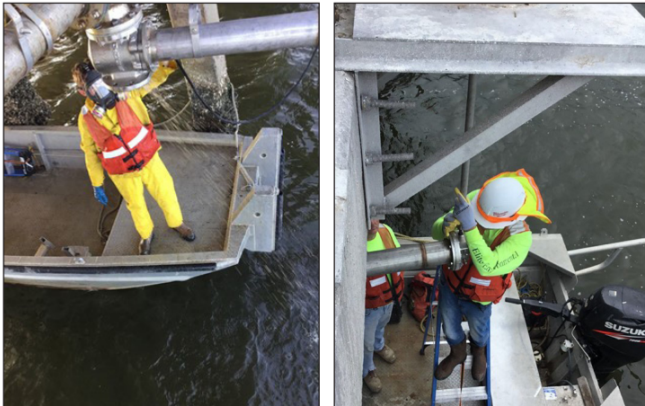
Crew members work from a floating platform to install a new custom fabricated valve operator and 4" plug valve at NAS Mayport, Florida.
